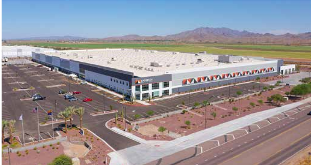
Andersen Window Manufacturing - Arizona
